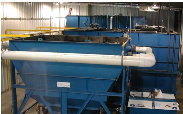
250 gpm clarifier used to treat acid mine drainage used as the water supply for a trout raising facility
