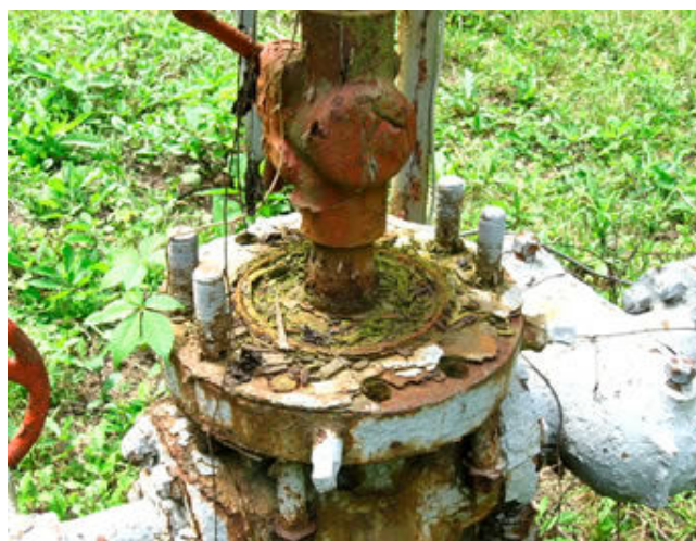
Photo 3. Severe corrosion at casing head and production pipe for the 47-039-02079 well in the Kanawha State Forest. Photo taken 29 August 2011.
