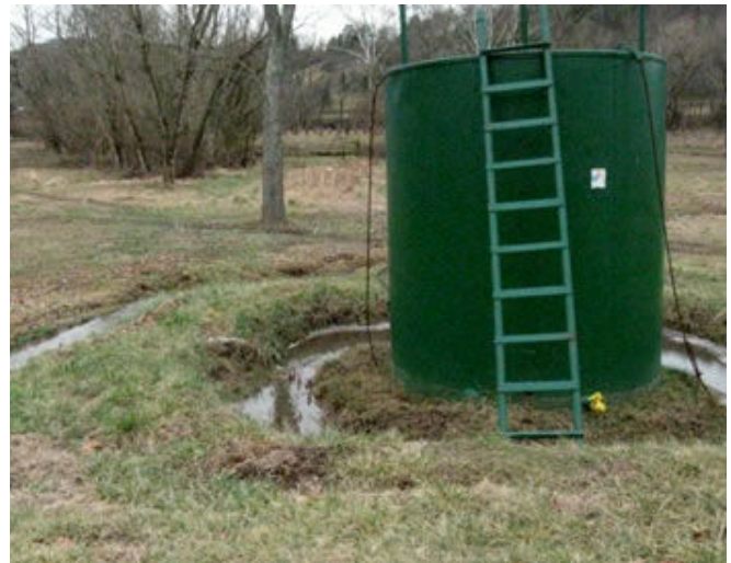
Photo 10. Moat type secondary containment for the 100 barrel tank at 47-079-00583. The tank's tethers hang unattached to the ground. The containment is partially filled with water and the dike is severely eroded on the side facing the permanent stream (on the left in the photo). Photo taken 12 January 2009.
