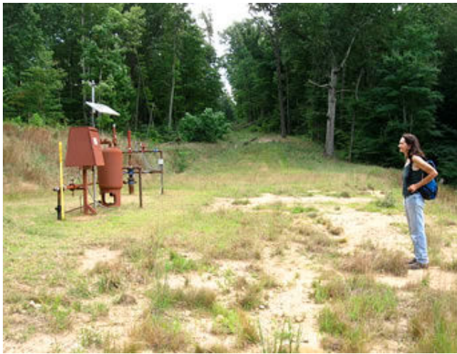
Photo 4. Well pad for 47-039-05772 which has a large expanse bare of vegetation between production equipment and edge of pad. This well site in the Kanawha State Forest had numerous signs of animal activity in the bare areas. Soil samples found elevated chloride. Photo taken 29 August 2011.
