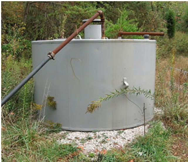
Photo 9. No secondary containment for the condensate storage tank exists at 47-079-00735. Photo taken 16 October 2008.
