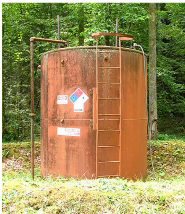
Photo 1. Condensate storage tank at 47-039-05500 well in the Kanawha State Forest. The overflow prevention device is visible at the top of the tank just to the right of the 10-foot high tank's ladder. Photo taken 29 August 2011.
