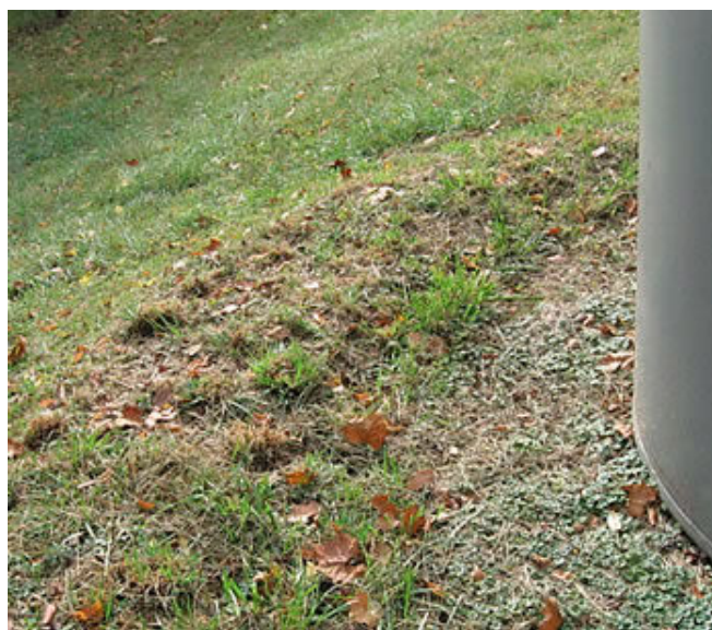
Photo 8. Inadequate secondary containment on river side of 47-079-00570 is no more than 8 inches high. The Pocatalico River is 47 feet downslope. Photo taken 16 October 2008.
