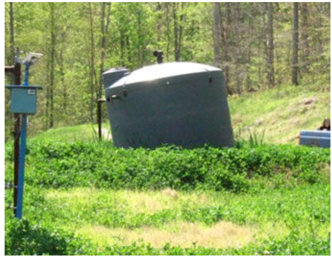
Photo 12. The large plastic condensate storage tank for 47-039-06155 floating within its water-filled secondary containment. Containment has a rainwater drain that appears to never have been used. Cattails are visible within the dike between the tank and the blue truck. Photo taken 30 April 2011.
