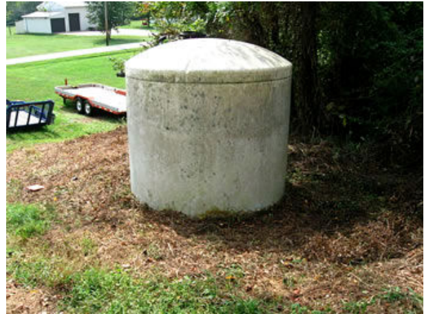
Photo 7. Large plastic condensate storage tank serving pipeline just north of Camp Virgil Tate Road. Tank doesn't have required secondary containment with rainwater drain. Pocatalico River is nearby to the south. Photo taken on 6 September 2012.
