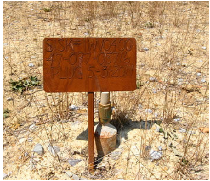
Photo 15. Improper monument for 47-097-03716, plugged in May 2011. Casing behind monument has smaller pipe set in cement with a closed vent on top. It's not clear why a plugged well would need a vent. Photo taken on 1 July 2012.
