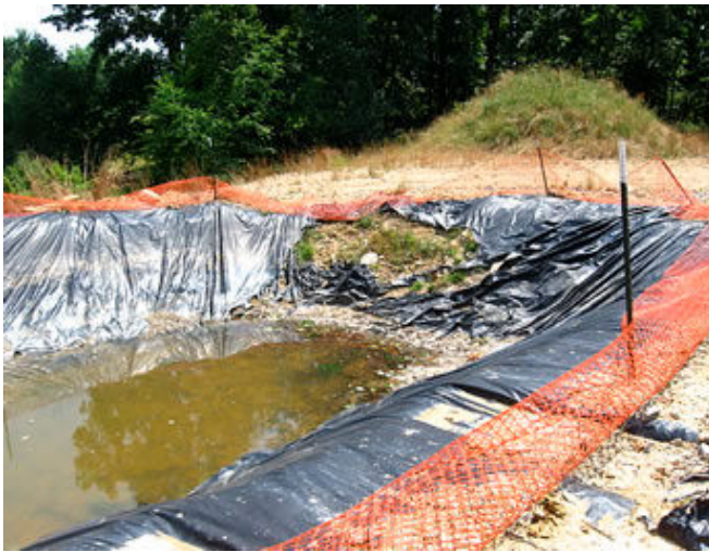
Photo 16. Smaller drill pit at 47-097-03716, a well plugged a year earlier. Liner is torn and fence is down even though cattle use field next to site. Pit appears to still retain fluid and cuttings. Photo taken on 1 July 2012.
