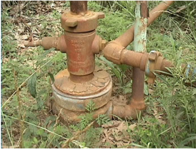
Photo 2. 47-079-00702 casing head with vent pipe on lower right hand side. Vent pipe (painted green) rises about 8 feet. Photo from video shot on 7 June 2012.
