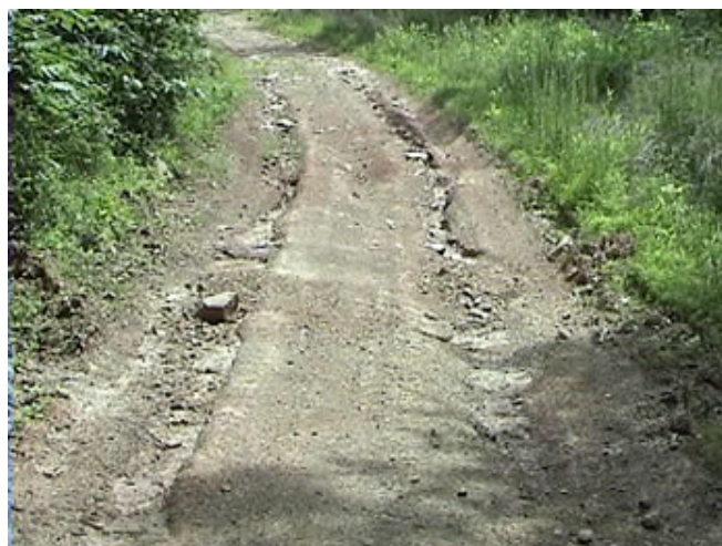
Photo 19. Well access spur from Long Road to 47-079-01314. Deeply rutted, the road's side ditches are filled with sediment. Photo from video shot on 7 June 2012.
