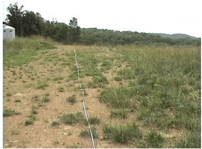
Photo 3. Barely vegetated pad for 47-079-01314. Tape measure follows line of exposed pit liner east of wellhead. See satellite photo of well site (photo 4) for comparison of location of pits in 2005. Photo from video shot on 7 June 2012.
