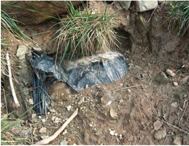
Photo 12. Buried liner and pit waste exposed in recent slip across pad of 47-079-01492. Photo taken on 12 October 2012.
