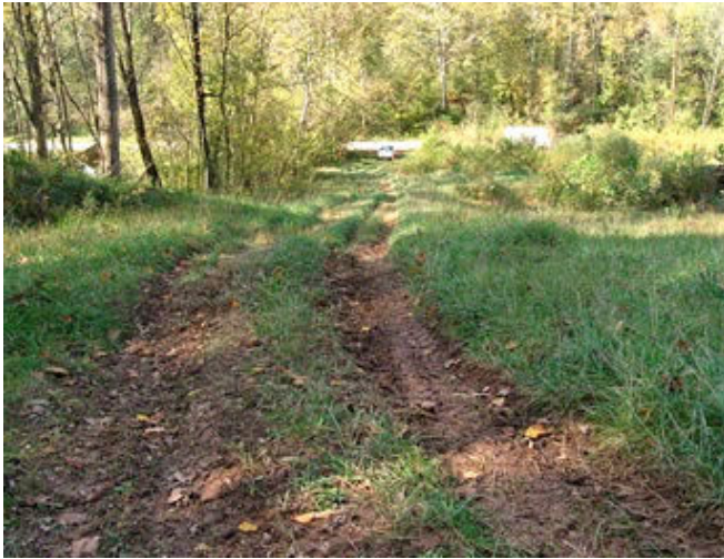
Photo 10. Steep grade for 47-079-01492 access road. Car is parked next to South Poca River Road. The Pocatalico River is just on the other side of paved road. Operator constructed a water bar part way up access road in 2009. This has not been maintained. Rain can wash sediment from access road directly into River. Photo taken on 12 October 2012.
