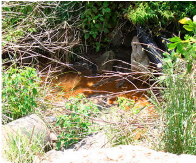
Photo 20. Sediment basin for culvert (not visible to the right). Photo was taken while standing on edge of newly constructed drainage ditch for the Tall Trees pad (47-097-03707 and 47-097-03708 horizontal Marcellus wells). Plastic pipes appear to carry drainage from cut slope to culvert. Photo taken on 1 July 2012.
