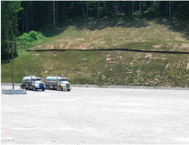
Photo 14. Portion of large gravelled pad at Tall Trees site (47-097-03707 and 47-097-03708 horizontal Marcellus wells). Steep cut slope is not adequately grassed. Two vac trucks at left in photo were waiting while another was removing condensate from one of the large storage tanks on the site. We were told that the tanks were emptied daily. Photo taken on 1 July 2012.
