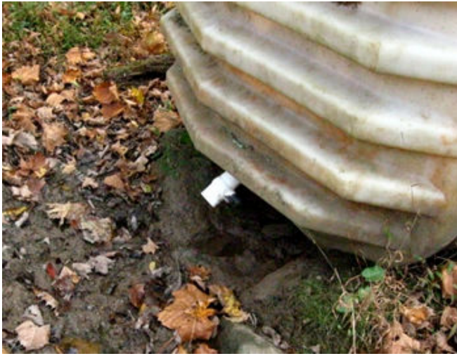
Photo 2. When we revisited 47-079-00615 in April 2013 we found the well producing. Fluid in the tank was slowly leaking from the valve at the bottom of the tank. The soil sample taken here had chloride at more than 641 ppm (the upper limit of our test method). Photo taken on 12 October 2012.
