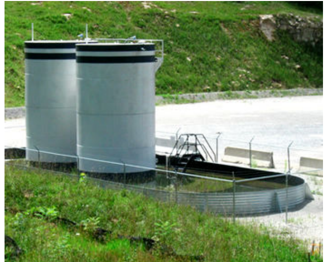
Photo 3. These two large storage tanks are at the edge of the Tall Trees pad in Upshur county (47-097-03707 and 47-097-03708 horizontal Marcellus wells). The containment would be adequate if it were not more than half full with standing water. Photo taken on 14 July 2013.
