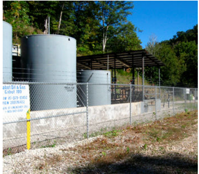
Photo 12. The tank battery at the UIC class 2 facility in the Amherst Plymouth WMA (47-079-01452). The 6 large tanks sit within cement lined secondary containment. The work area is covered with a metal roof toward the middle right of the photo. Photo taken on 6 April 2013.
