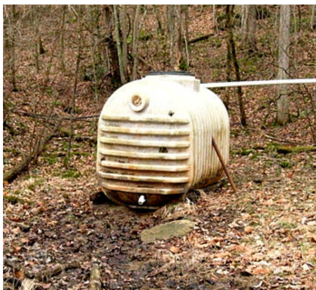
Photo 17. This is what the inspector in the Office's report wrote about 47-079-00615: "double walled tank looked o.k." The tank is leaking at the valve at the bottom and requires replacement or repair. The single wall tank requires secondary containment. Photo taken on 26 February 2009.
