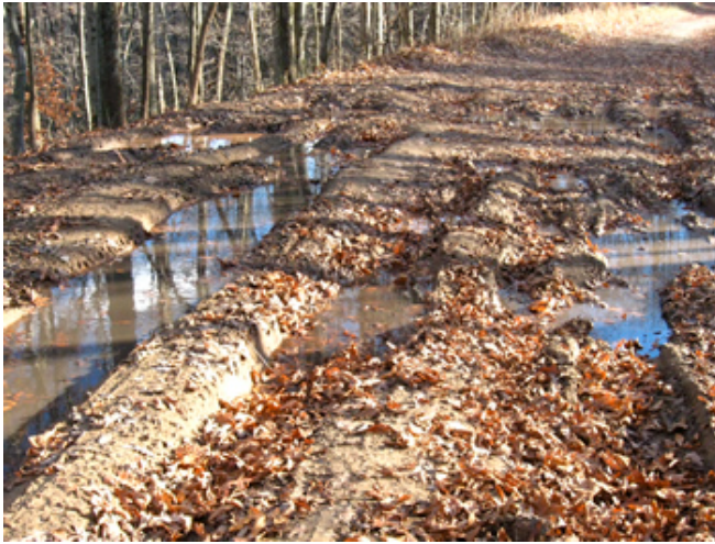
Photo 21. This photo shows the main well access road for a number of gas wells (what we call the Long Road). This spot is just north of 47-079-00702 and is deeply rutted. The Office's report found no issues with the road – "drains in good condition." Photo taken on 18 November 2013.
