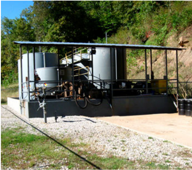
Photo 11. The UIC class 2 well facility in the Amherst Plymouth WMA (47-079-01452). The cement unloading area (with curb) is in the right foreground. The work area with pump and filters is in the middle ground. A steel grate covers the whole work area platform so that any spilled fluids go into a sump. The tank battery within a cement lined secondary containment is visible in the background. Photo taken on 6 April 2013.
