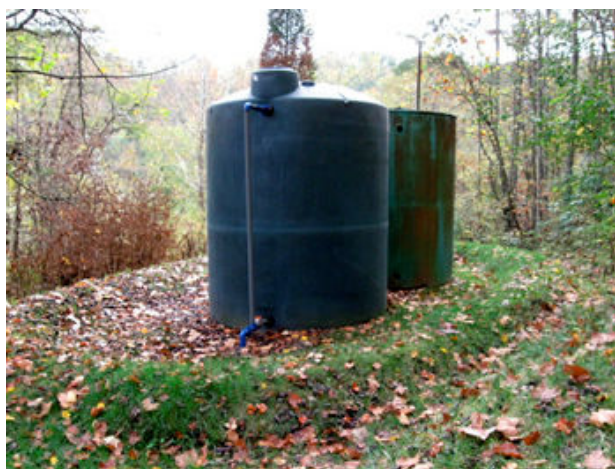
Photo 1. Tanks at 47-079-00746. The steel tank behind the large plastic tank has large holes. Containment dike has eroded on river side (left in photo) so that containment no longer is adequate. Photo taken on 16 October 2008.
