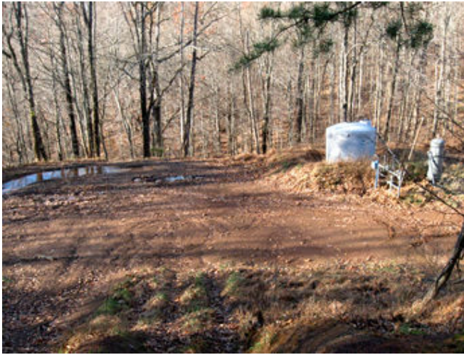
Photo 18. This provides a view of the mostly bare pad for 47-079-00702. The bare pad extends an equal distance to the left of the photo. Vegetation on the pad surrounds the well equipment only. The inspector wrote of this site in the Office's report: "site looked good with grass/vegetation growing." Photo taken on 18 November 2013.
