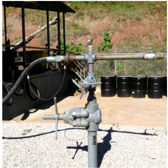
Photo 9. The UIC class 2 wellhead at 47-079-01452. The black pipe to the left carries fluid to the well. There's a pressure gauge on top of the wellhead. The annulus pressure gauge is hidden by the well in this photo. The cement unloading pad is visible behind the wellhead. The pad is sloped toward the work area and toward the sump under the steps behind the wellhead. Photo taken on 6 April 2013.
