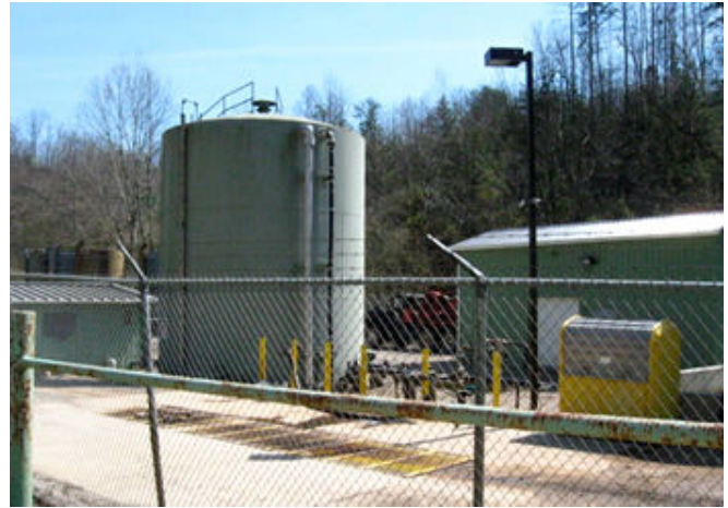
Photo 7. The large tank at UIC class 2 well 47-039-02210 next to Tupper's Creek holds 57,000 gallons. It has a flammability warning posted. There is no visible secondary containment. The unloading pad is in the foreground. The yellow grid appears to be grates covering a sump. Photo taken on 6 April 2013.
