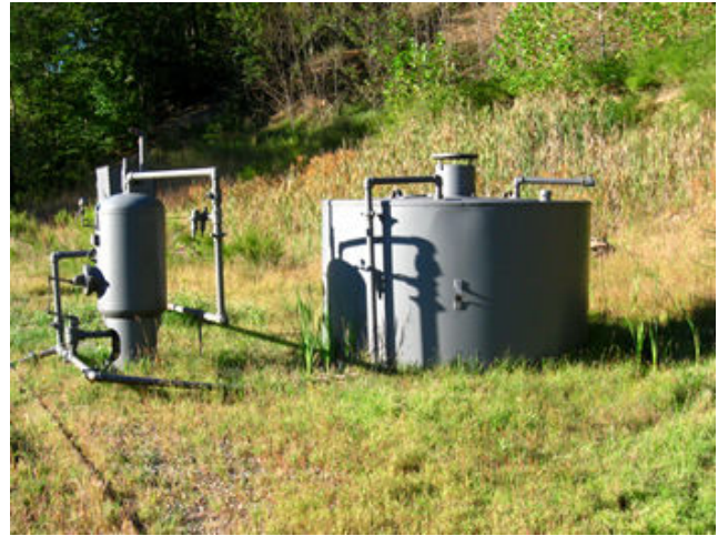
Photo 5. Tank and separator for 47-079-01324. The tank does not have required secondary containment. Photo taken on 23 September 2013.
