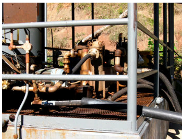
Photo 15. The work platform at the UIC class 2 facility in the Amherst Plymouth WMA (47-079-01452). The cement walled platform is covered with a grate so spilled fluids go into a sump. The black pipe in the foreground goes to the injection wellhead. Photo taken on 6 April 2013.
