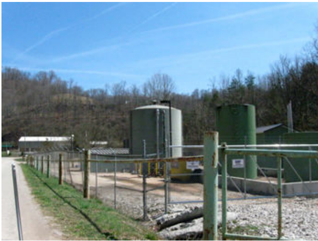
Photo 8. The UIC class 2 facility next to Tupper's Creek (47-0039-02210). The containment with two smaller tanks is in the right foreground. In the center of the photo is the 57,000 gallon tank. Utility buildings and the injection well are behind the large tank. The site is well secured with fencing and locked entrance gates. Photo taken on 6 April 2013.
