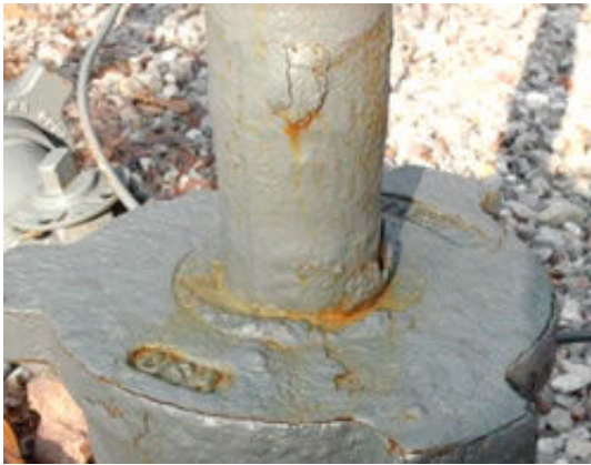
The corroded production pipe at 47-039-02026 has been painted but is still in need of replacement.
