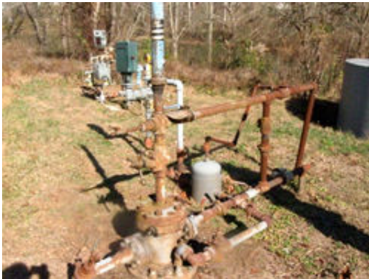
Corroded metal at 47-079-00570 needs to be painted.
